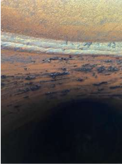
ONGUARD Product Results (Ceiling of Railcar with Asphalt Residue)
